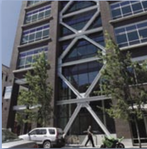
WILLAMETTE UNIVERSITY PORTLAND CENTER – PORTLAND, OR (PEARL DISTRICT)
