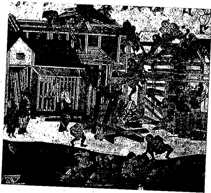
Construction crews build merchant houses in the Nibonbashi area
